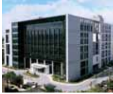
Taoyuan Technology Center (Green Building)
